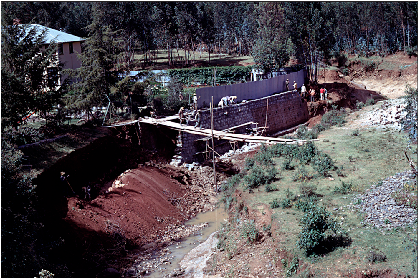
Building the Wall
