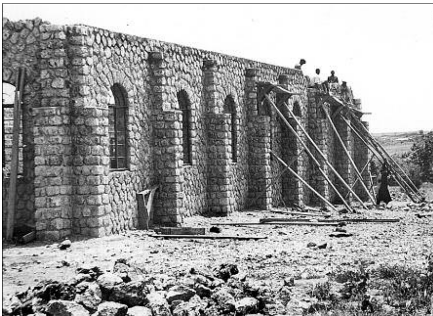
Kirk Memorial Chapel under construction, 1953.
