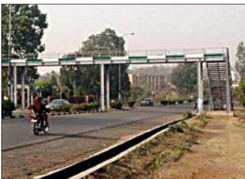
Hillcrest crosswalk. A monstrosity built to help folks over the constantly streaming traffic on Old Bukuru Road
