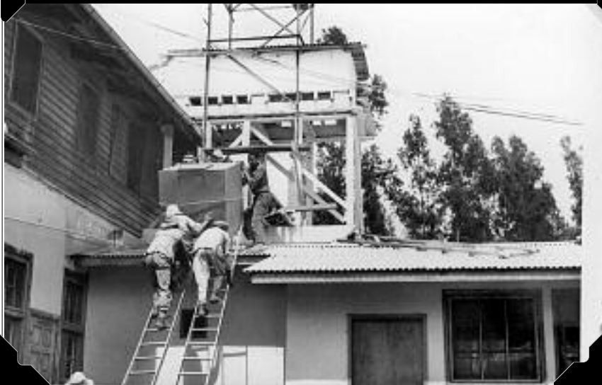
Raising a new water tank above the kitchen.
