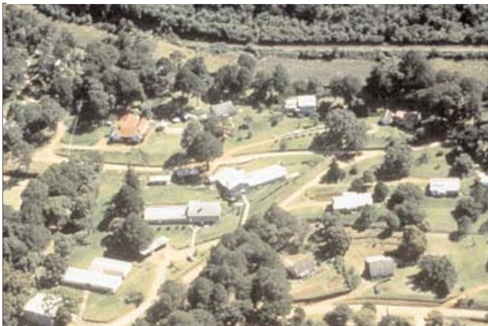
The upper part of RVA campus with railway tracks
